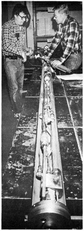
DEEP STEAM instrumentation package, with hoses, one-way valves, filters, temperature sensors and electronics, is assembled in the welding shop. The package, which monitors pressures and temperatures, will be mounted directly above the steam generator unit at the bottom of the oil well. It is designed to operate continuously in a 500°F environment. John James and Dave Paul (both 2166) assemble the package prior to its being sealed and welded.
